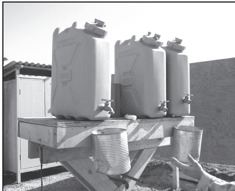
Figure 5-10. Improved handwashing facility
